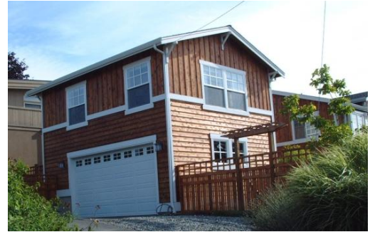
An ADU above a garage, Kirkland
