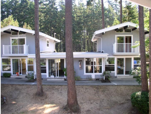
Chalet Apartments, St. Andrew's Housing, Bellevue
